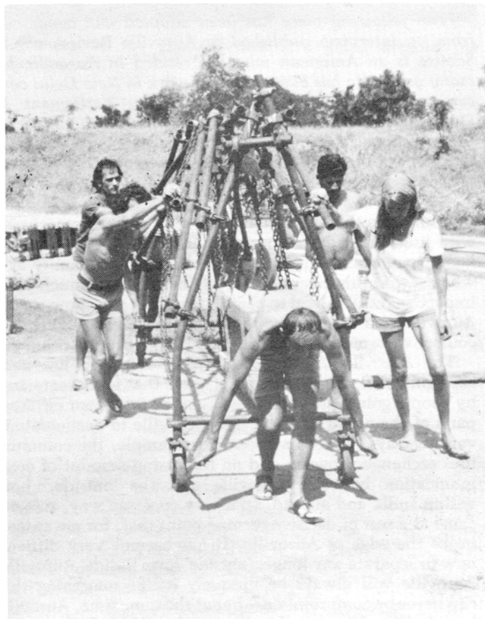
Aurovilians carrying sections of precast forms for Matrimandir
